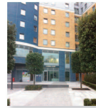
BSA London Meeting Room External View
