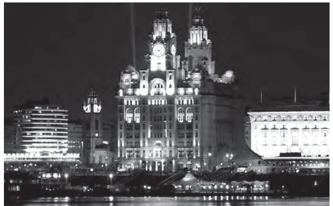
THE LIVER BUILDINGS, LIVERPOOL
